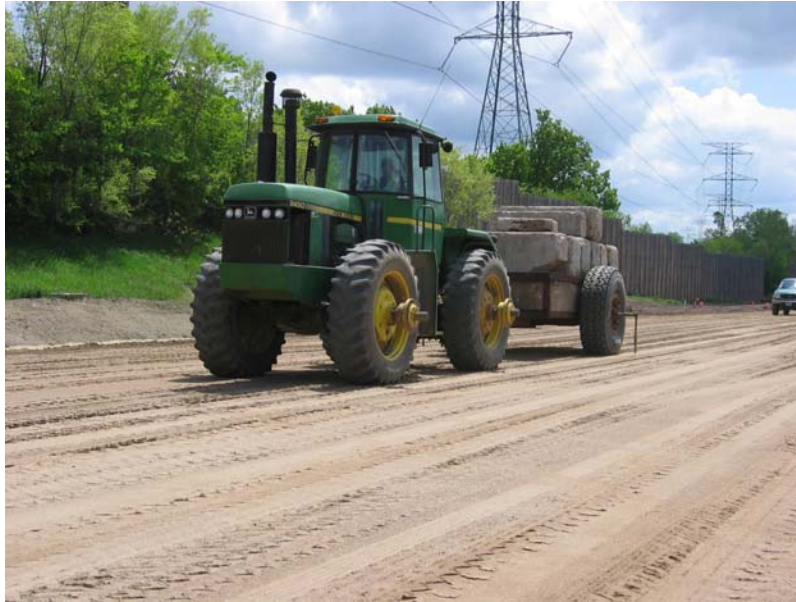
Figure 1.3. Test rolling a compacted subgrade.
