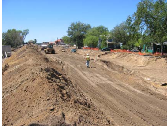
Figure 2.1. Construction of Highway 10 in Staples, MN.
