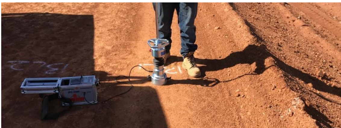
Figure 2: LWD testing of lime treated general fill using the Zorn device 13/12/19
