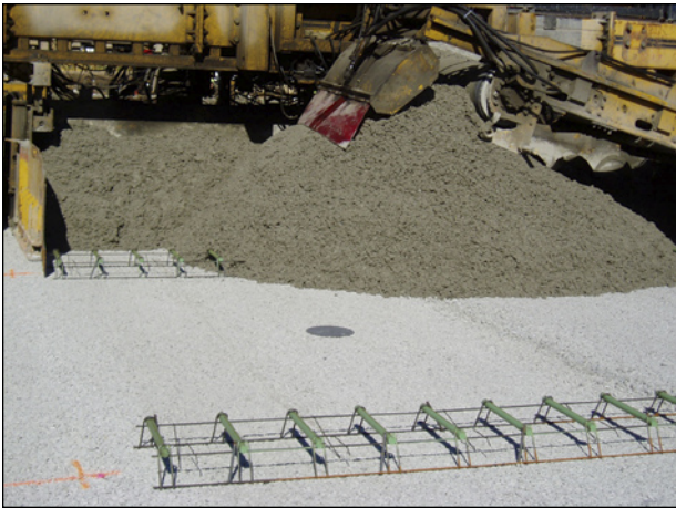
Figure 2. Preplacement of a reflector on the base.
