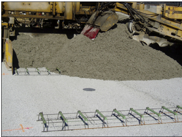
Figure 2. Preplacement of a reflector on the base.
