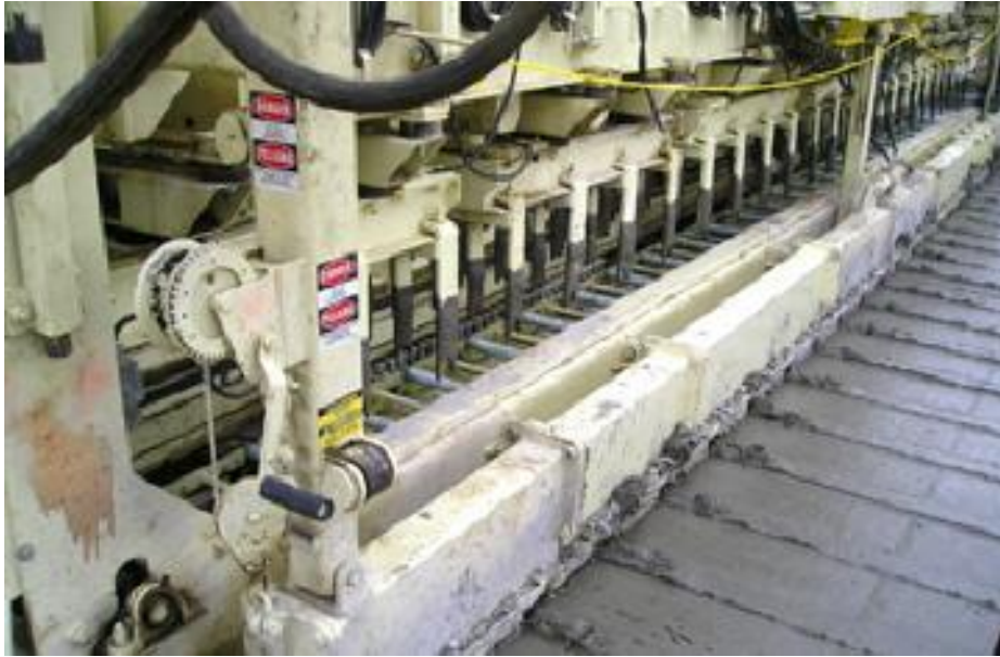
Figure 1.2 Dowel Bar Inserter (DBI)
