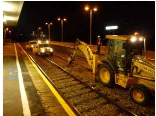
Figure 2: Test pit excavations
