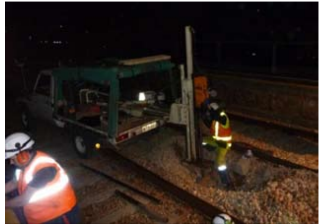
Figure 5: Drilling into rail formation
