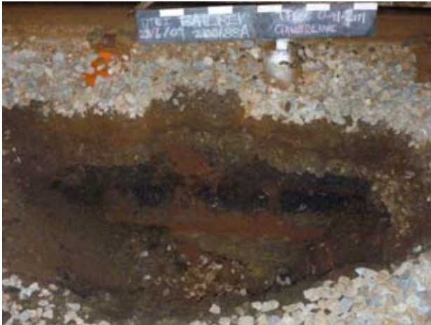
Figure 4: Layers of ballast, sub-ballast, cinders, fill and subgrade
