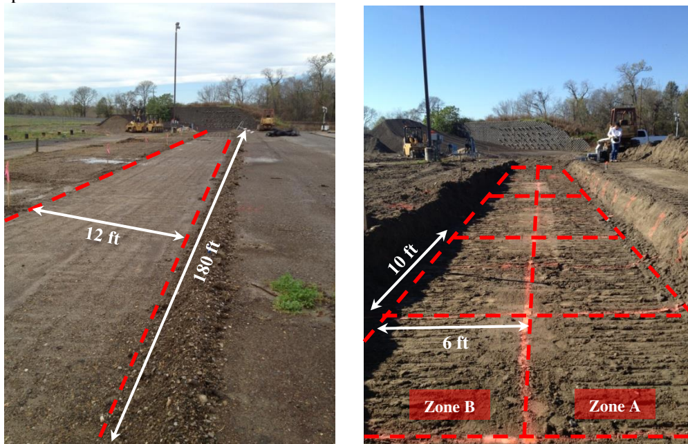
Figure G.2.2 – Typical LTRC Test Section
