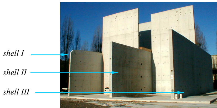
Fig. 11 Structure on which method has been tested.
