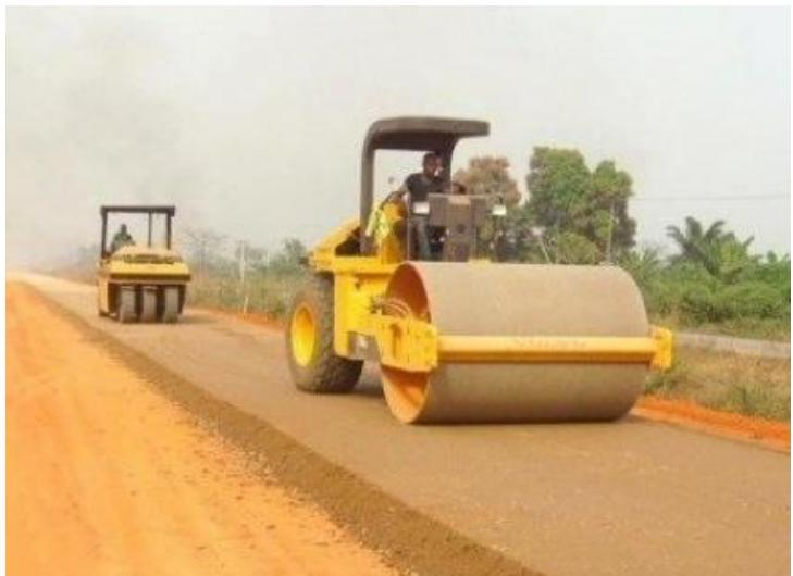
The **mechanical behavior of the pavement layers** is by the nature of the materials, the thickness of the layers and **the level/quality of compaction**.
