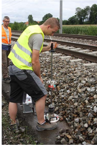
Figure 20: A LFW being used on an asphalt trackbed layer in Austria. (ÖBB – Austrian Federal Railway)
