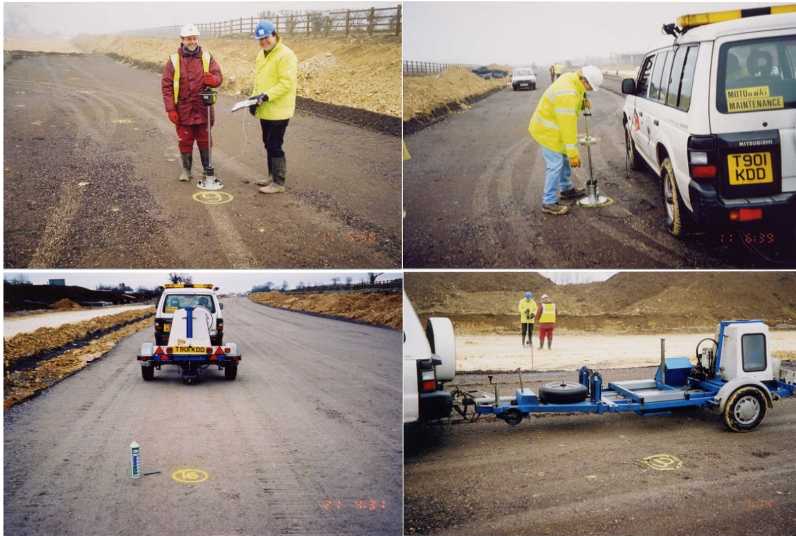
Figure 1. Test at sub-formation level comprises FWD, Prima and GDP testing at the same location as FWD
