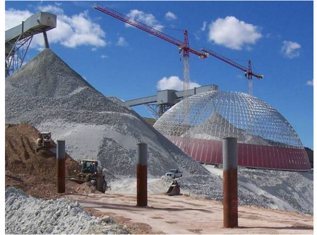
Figure 8. Construction of Coarse Ore Stockpile Dust Covers
