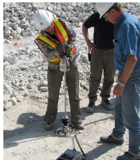
Figure 9. Testing of Coarse Fill with the LWD
