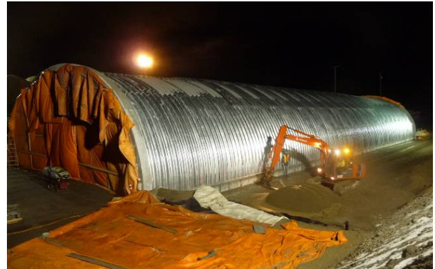
Figure 6. Night Time Construction at the Multiplate Underpass
