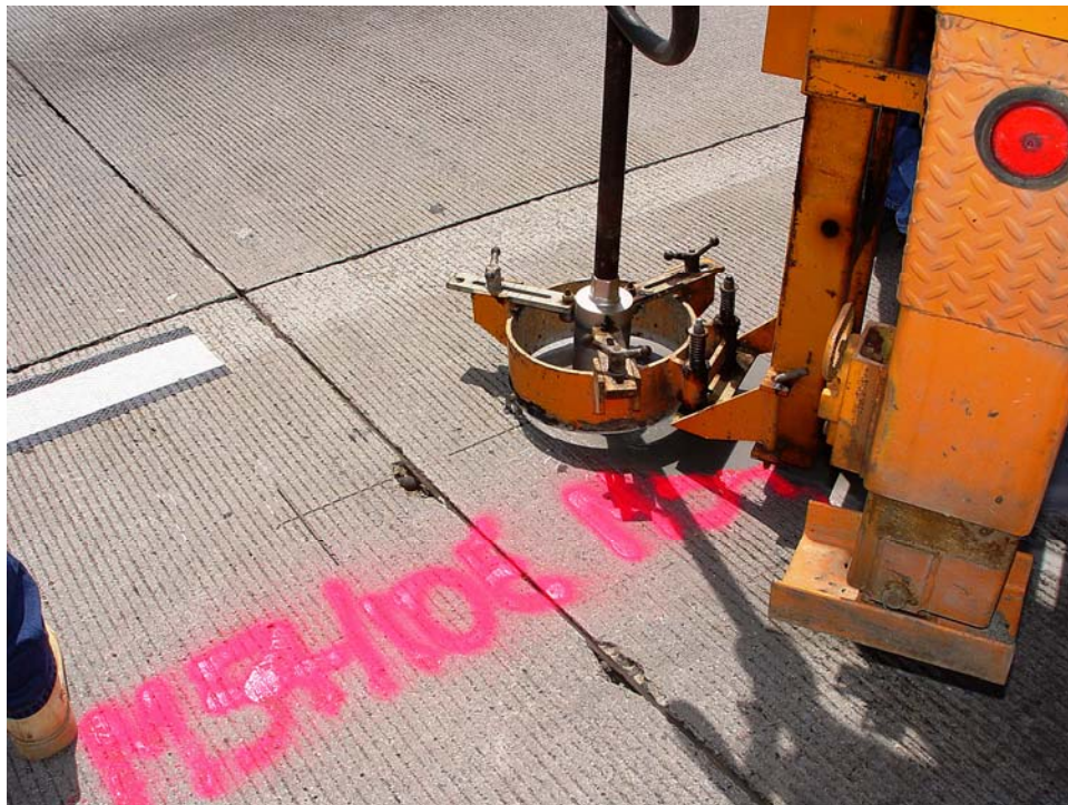
Figure 12. Field Coring Operation Near Joint 54 on I-66
