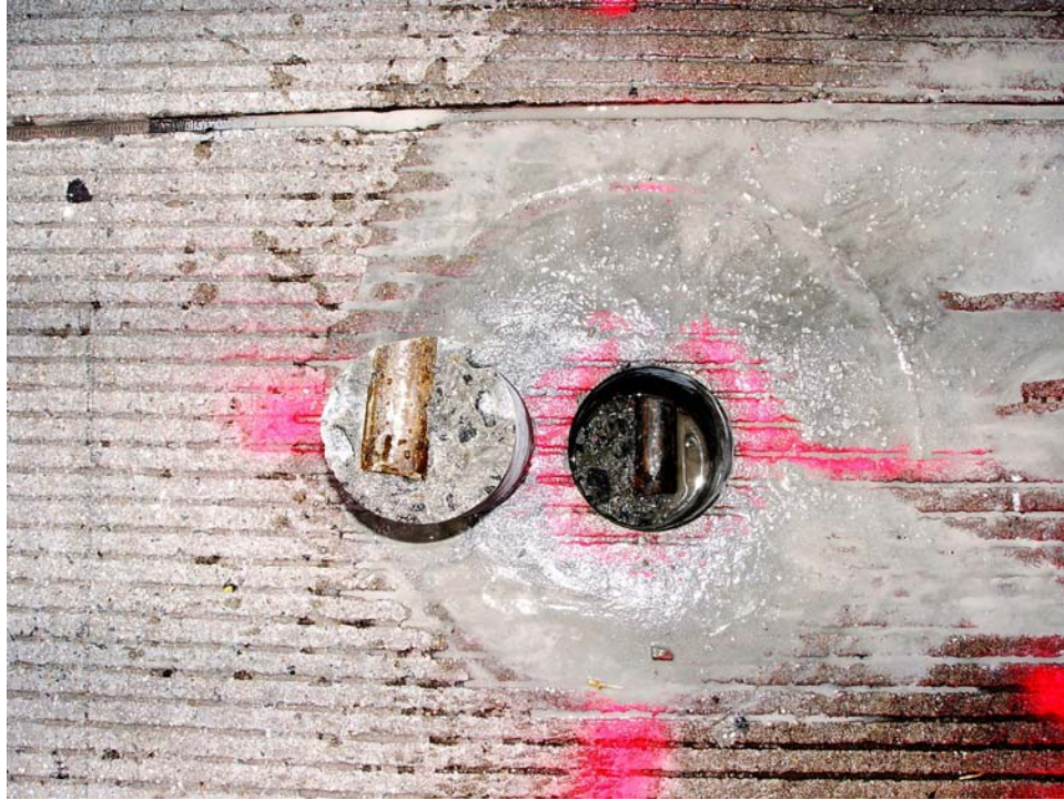
Figure 13. Field Core and Dowel Bar Near Joint 43 on I-66
