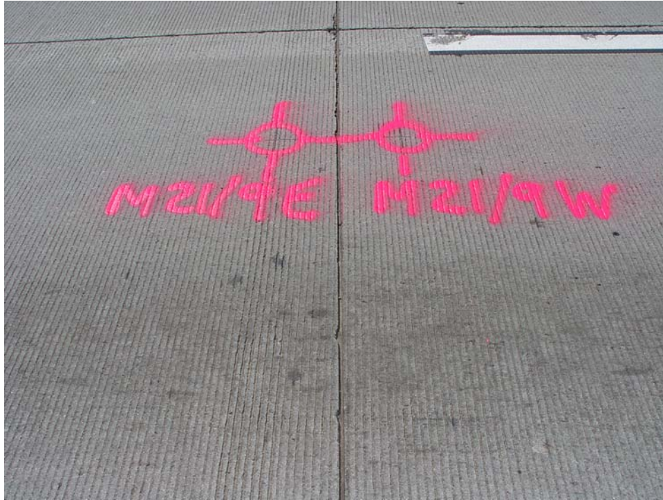
Figure 11. Field Marking of Dowel Bar Near Joint 21 on I-66
