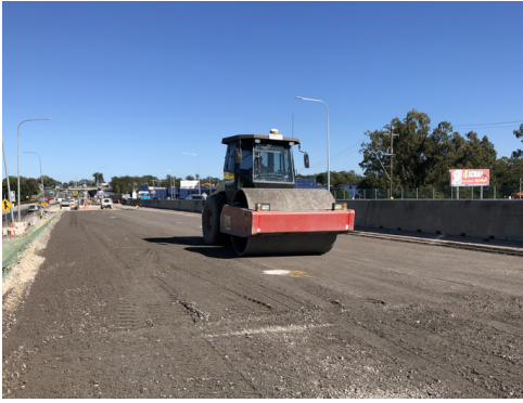
Fieldwork demonstration of Intelligent Compaction in Queensland
