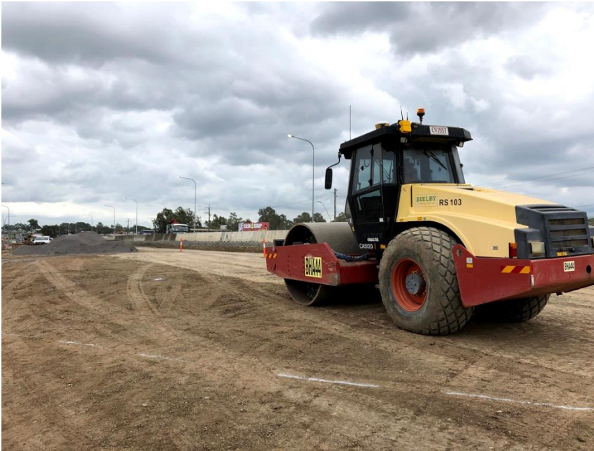
Figure 3.3 A Dynapac smooth drum roller installed with IC technology
