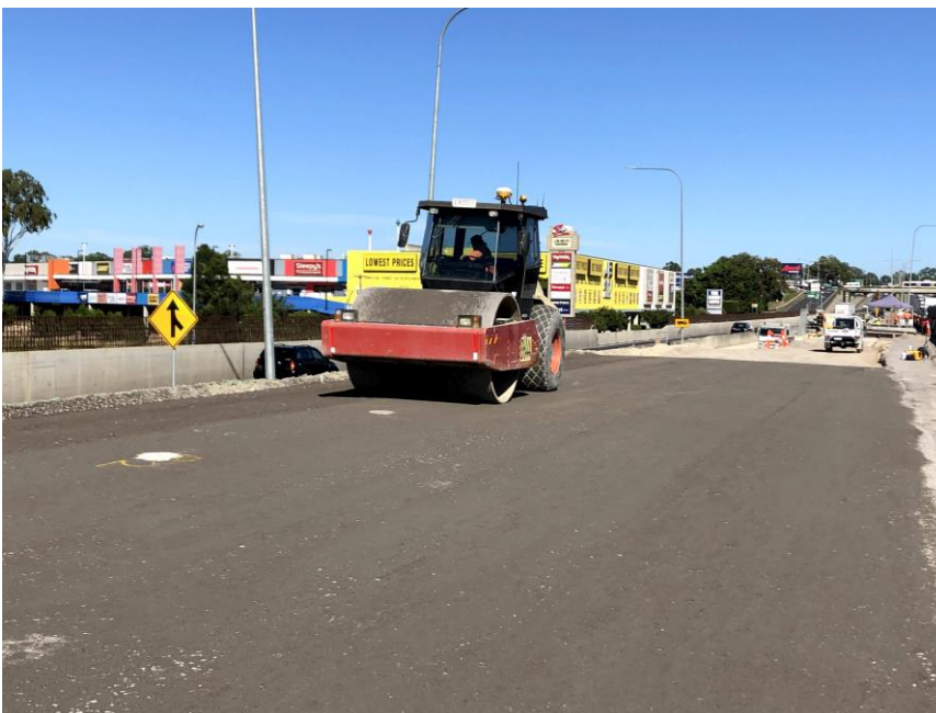
Figure 3.10 IC roller compacting a cement modified layer
