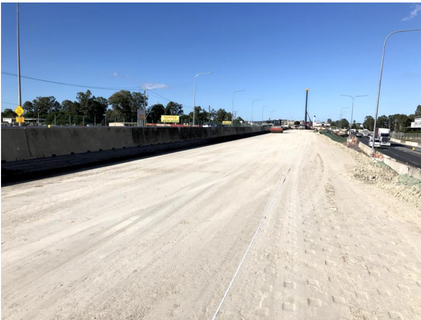
Figure 3.8 A subgrade area ready for IC pre-mapping
