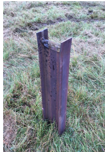
Figure 5. Pile damaged during trial installation
