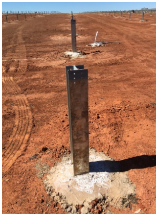
Figure 6. Piles installed after pre-drilling
