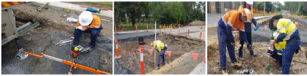
Figure 2. Subgrade preparation and testing
