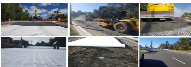
Figure 3. Installation of pressure cell, geocomposite, geogrid, gravel and asphalt
