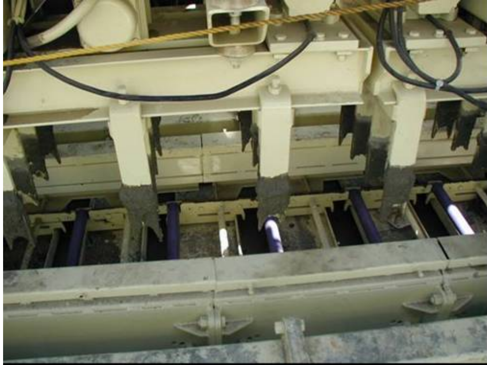
Figure A.5. Placement of dowels using a DBI.
