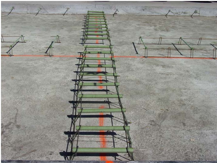
Figure A.4. Placement of dowels in dowel baskets prior to paving.
